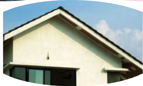
UCO Vistabord used as external soffits and wall cladding
